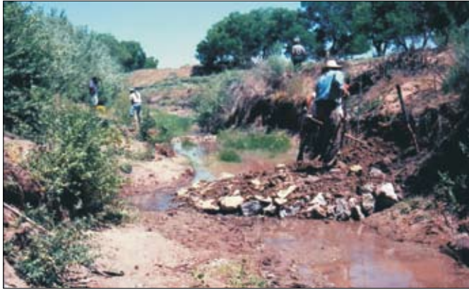
A newly installed rock baffle at Hubbell Trading Post, AZ, June 1997.
