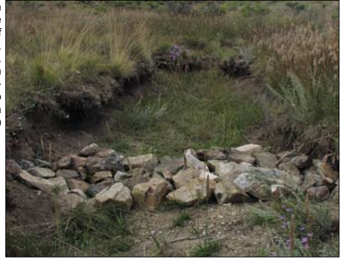
One rock dam on a side drainage of Holman Creek, Valle Vidal, Carson National Forest, NM (Photo by Tamara Gadzia.)
