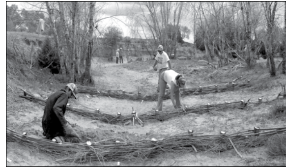
Workshop volunteers build a wicker weir on Largo Creek, Williams Ranch, Quemado, NM. August 2004. Photo by Tamara Gadzia.
